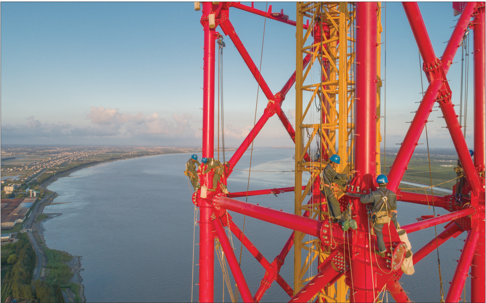
On 7 August, the first main tower of 500 kilovolt Haimen Dongzhou – Shanghai Chongming electricity transmission project Yangtze River north channel major crossover reached 180 m in height. The technicians accelerated construction under high temperature, to complete the energy main artery as soon as possible. Photo by Huang Hai
